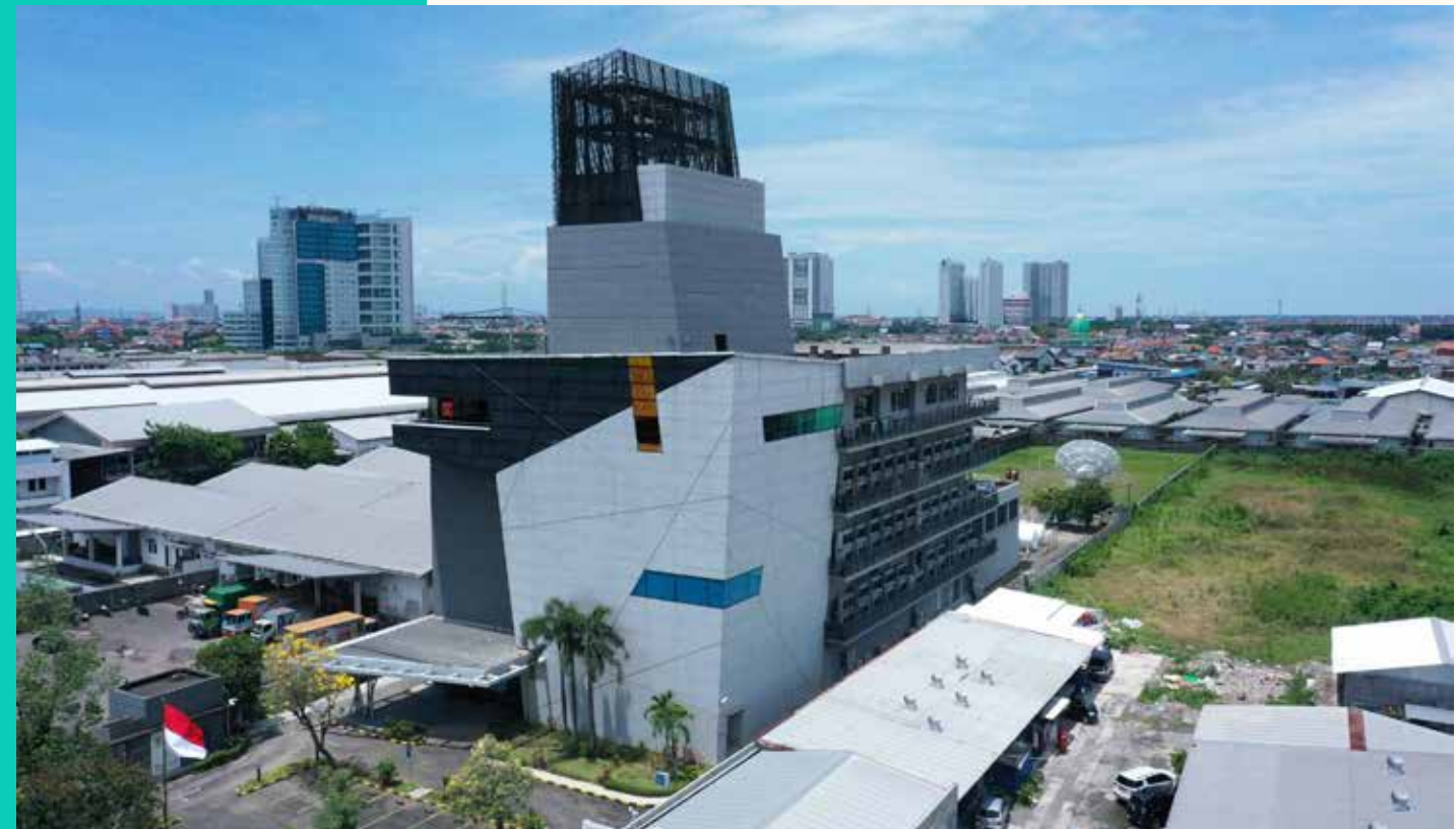
PDG's JB1 Data Center in Jakarta, Bintaro
